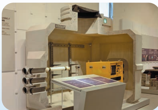
Manhole to pass through communications cable (model)
